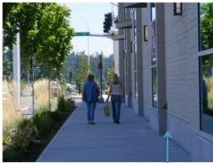
Simple concrete base differentiated from brick veneer
