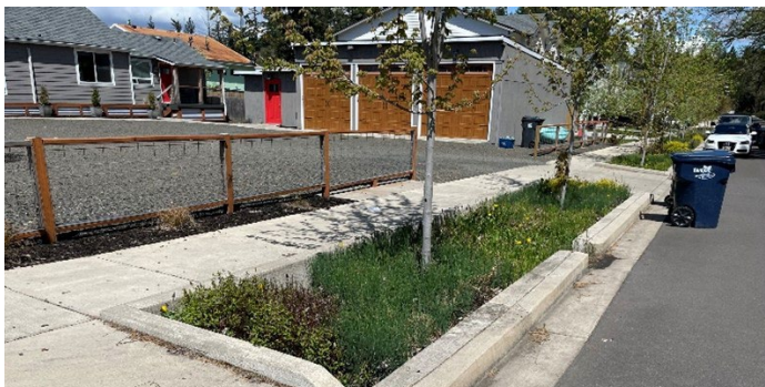
FIGURE 6. AN EXISTING BIOSWALE TO FILTER STORMWATER ON JAMESON WAY. PHOTO: DLA
