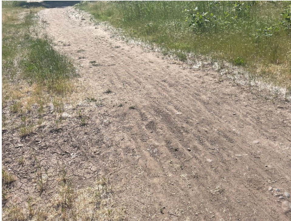
FIGURE 38. EXAMPLE OF WASH BOARDING FROM WATER DAMAGE. SOURCE: DLA
