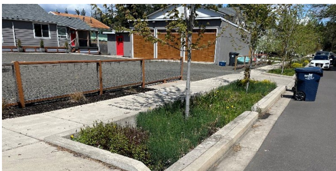
FIGURE 6. AN EXISTING BIOSWALE TO FILTER STORMWATER ON JAMESON WAY. PHOTO: DLA
