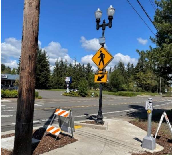
Rectangular rapid flashing beacons along Territorial Hwy making crossing safer and more comfortable
