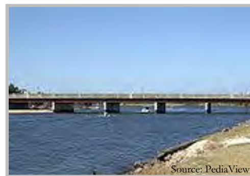
Example of causeway built on piers
