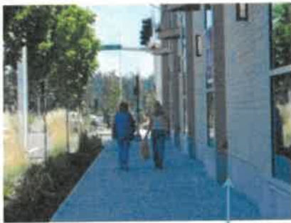
Simple concrete base differentiated from brick veneer
