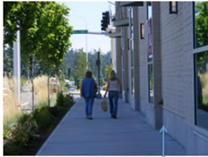
Simple concrete base differentiated from brick veneer
