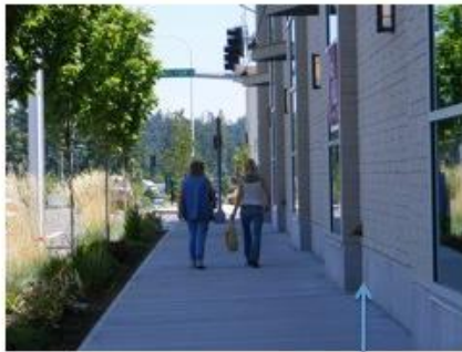
Simple concrete base differentiated from brick veneer
